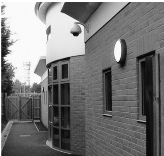
Image 16: Window to circular court
