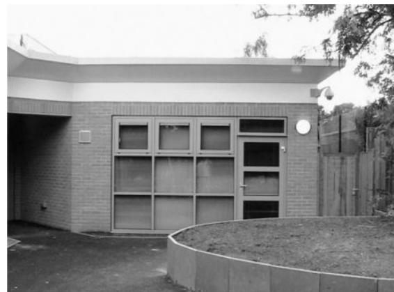
Image 18: Classroom picture window
